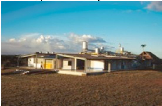
Self-sufficient hospital of Las Gaviotas, Colombia. Photo © ZERI, 2000
