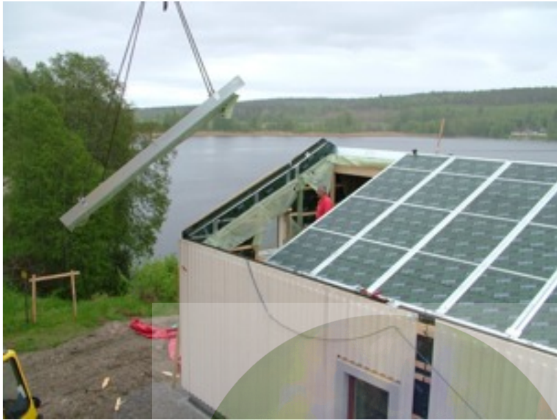
A prefabricated house with foundations, walls and roof made from recycled glass. Designed and constructed by Åke Mård in Sundsvall, Sweden. Photo courtesy of Åke Mård of MRD (Sweden)
